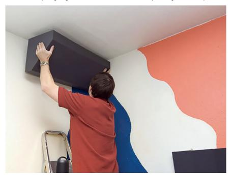
The boundary between the ceiling and the walls is just as much of a corner as the meeting of two walls, in acoustic terms. A foam bass trap intended for corner mounting can be mounted at ceiling height, if necessary, where it will be just as effective, without having to give up any floor space. You will need rather more than just this one, though!
